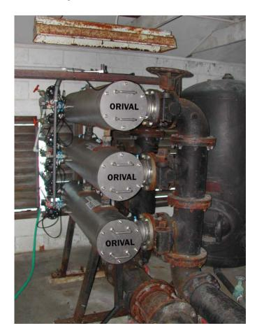
Figure 2. Three High Performance Stainless Steel Filters
